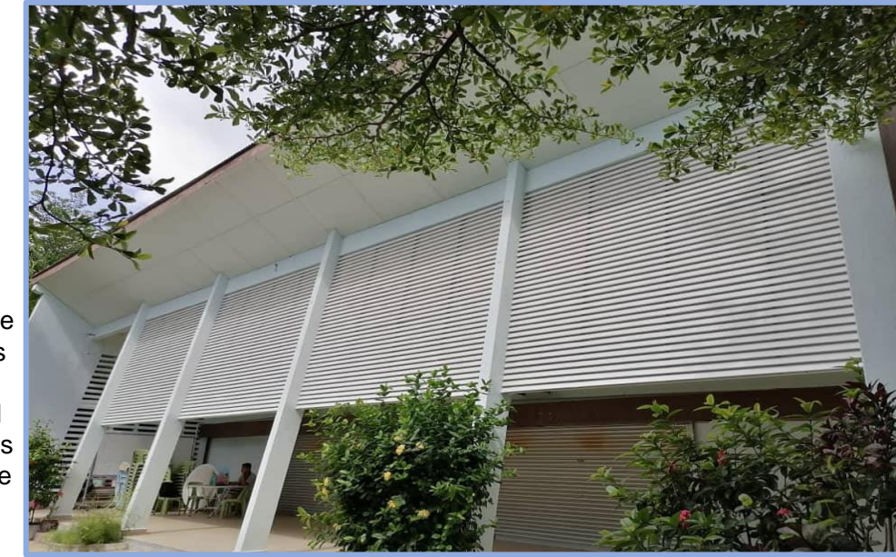
A renewed front of Christian Convention Center which was completed during MCO.
